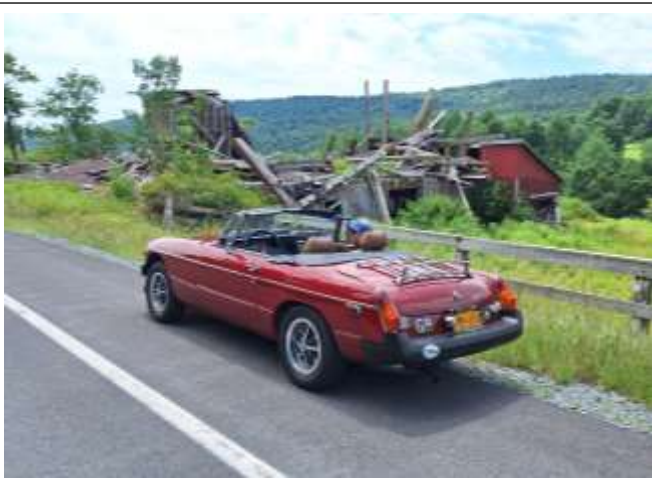
Destination #28 – Dilapidated Derelict Run-down Barn - Goodwin
