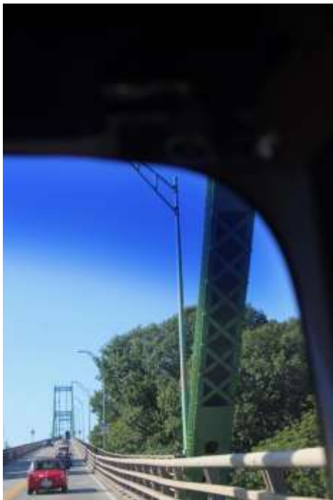
3 The Barlows head over the bridge
